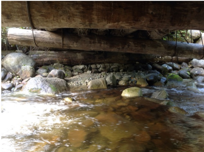
Left Bank Abutment when facing downstream
